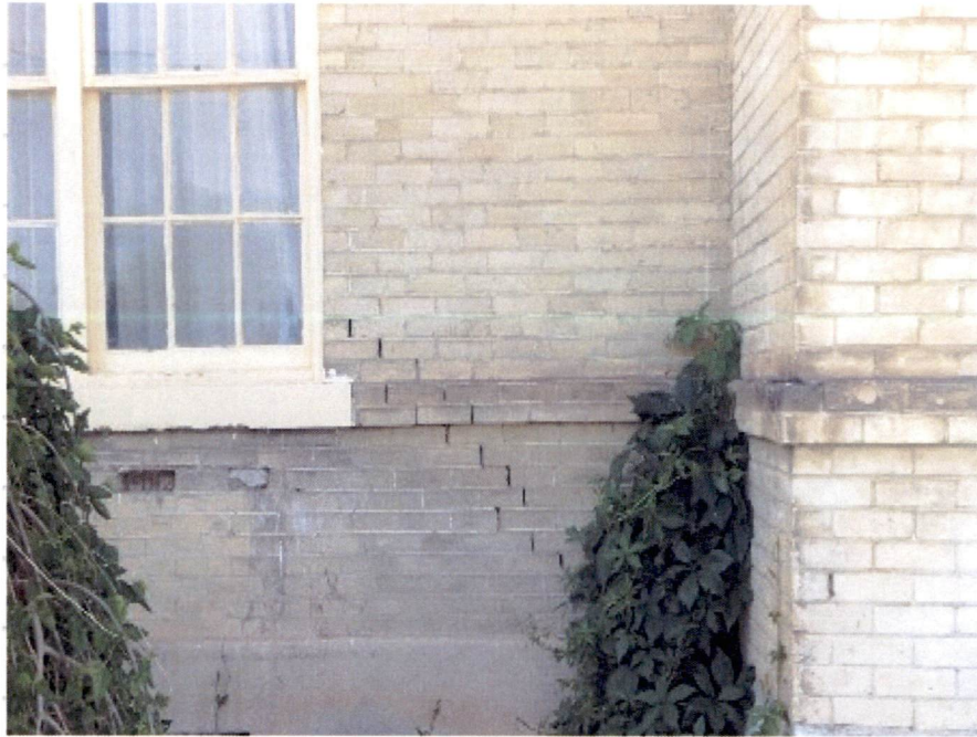
Figure 7- West exterior with Cracks
