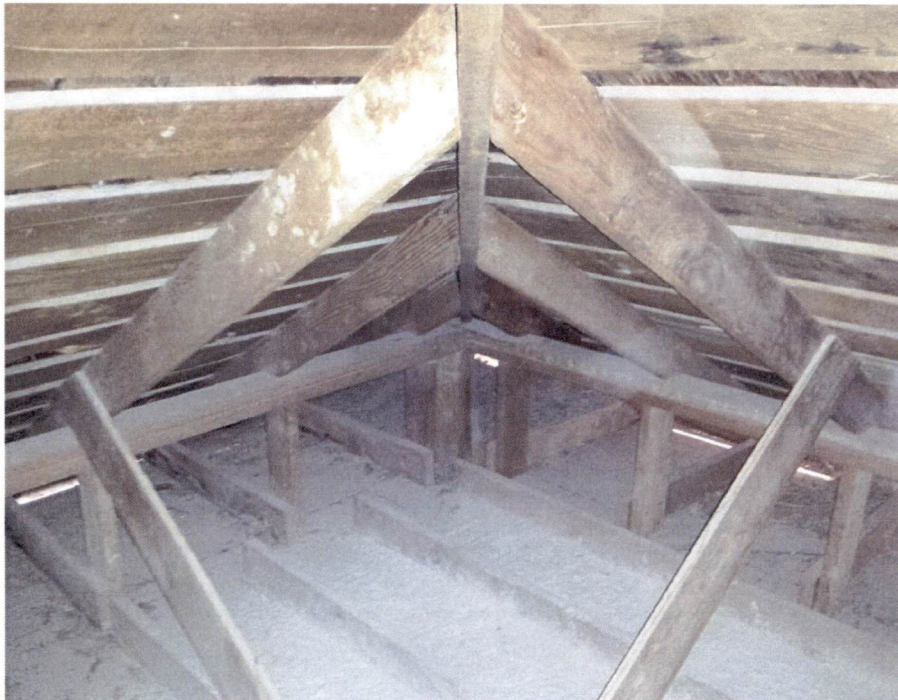
Figure 12- Framing support for tower
