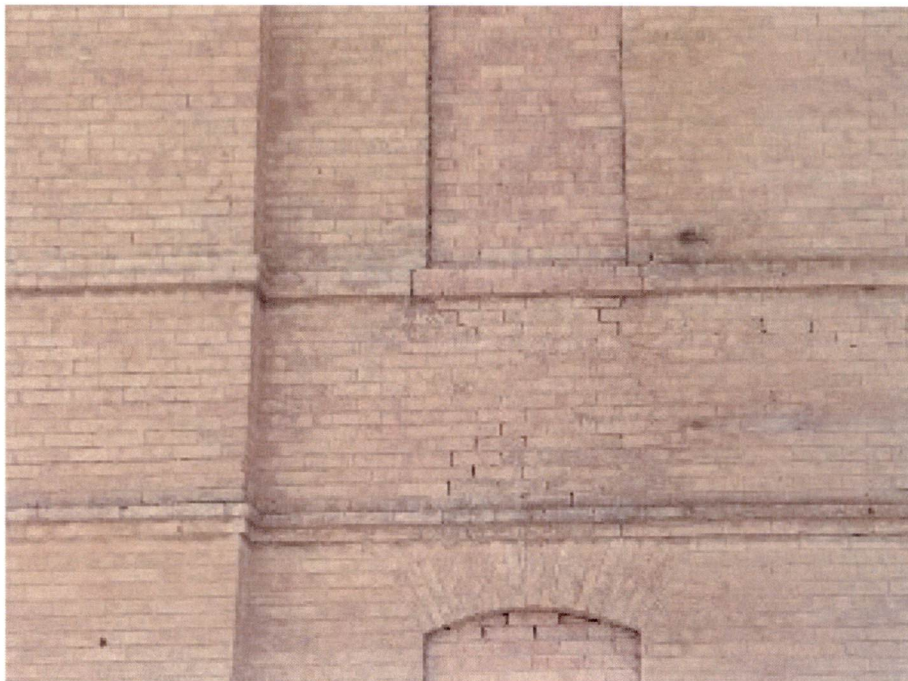
Figure 4- North side showing cracks
