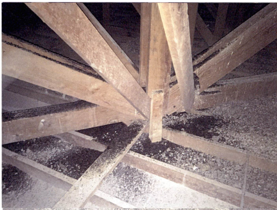
Figure 14- bat guano in the attic
