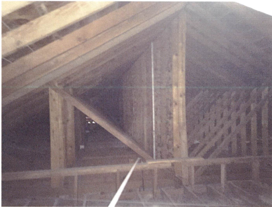
Figure 13- Roof framing
