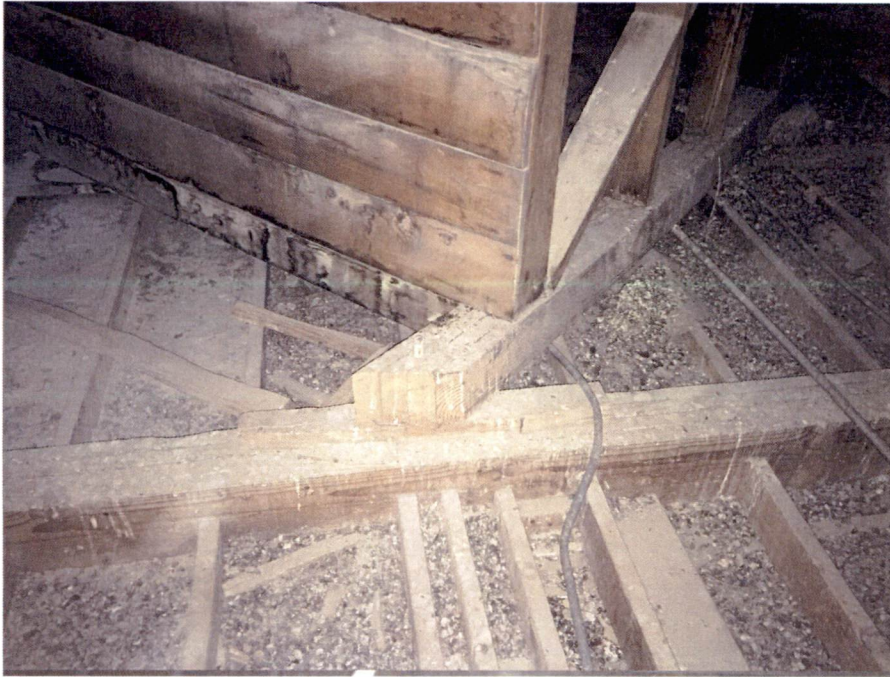
Figure 13 - Support base for tower
