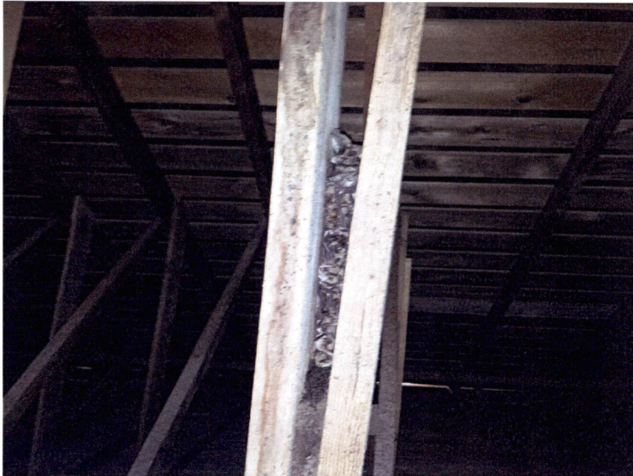
Figure 10- Framing support for tower
